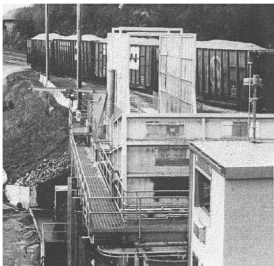
FIGURE 2.20 Rail cars ready to be unloaded. They will be tipped back on the special platform to discharge their contents. Over six cars per hour can be unloaded by this method.
